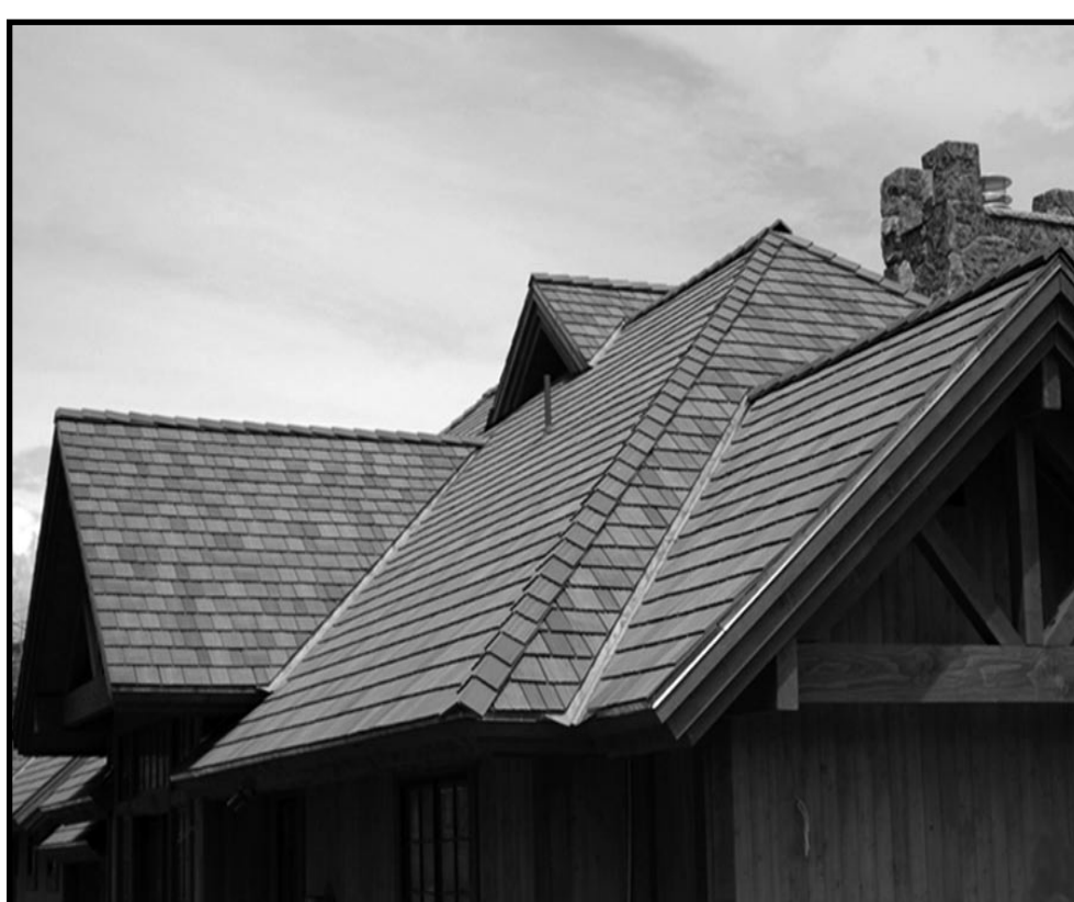
Synthetic Shake roofing tiles resist fire, severe weather, impact, and insects. The durable tiles have a 50-year warranty.
